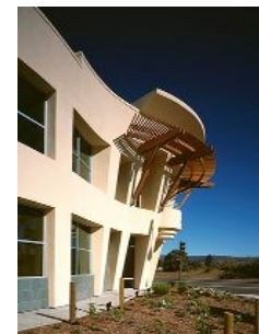
Corner detail of Napa Community Bank Building, Napa, California.
