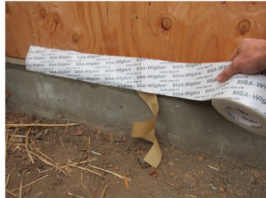
Photo 2. Tape wall sheathing to concrete foundation for continuity of air barrier
