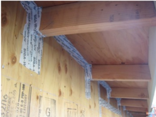
Photo 1. Tape wall sheathing to roof sheathing for continuity of air barrier
